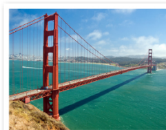
Golden Gate Bridge
